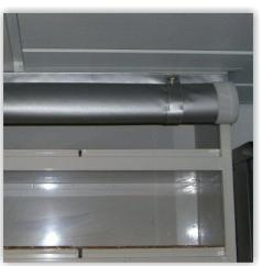
Mulitple coatings of silicone on woven glass fabric ensure it is strong, yet flexible enough to be fabricated into high performance permanent fit smoke curtains.
